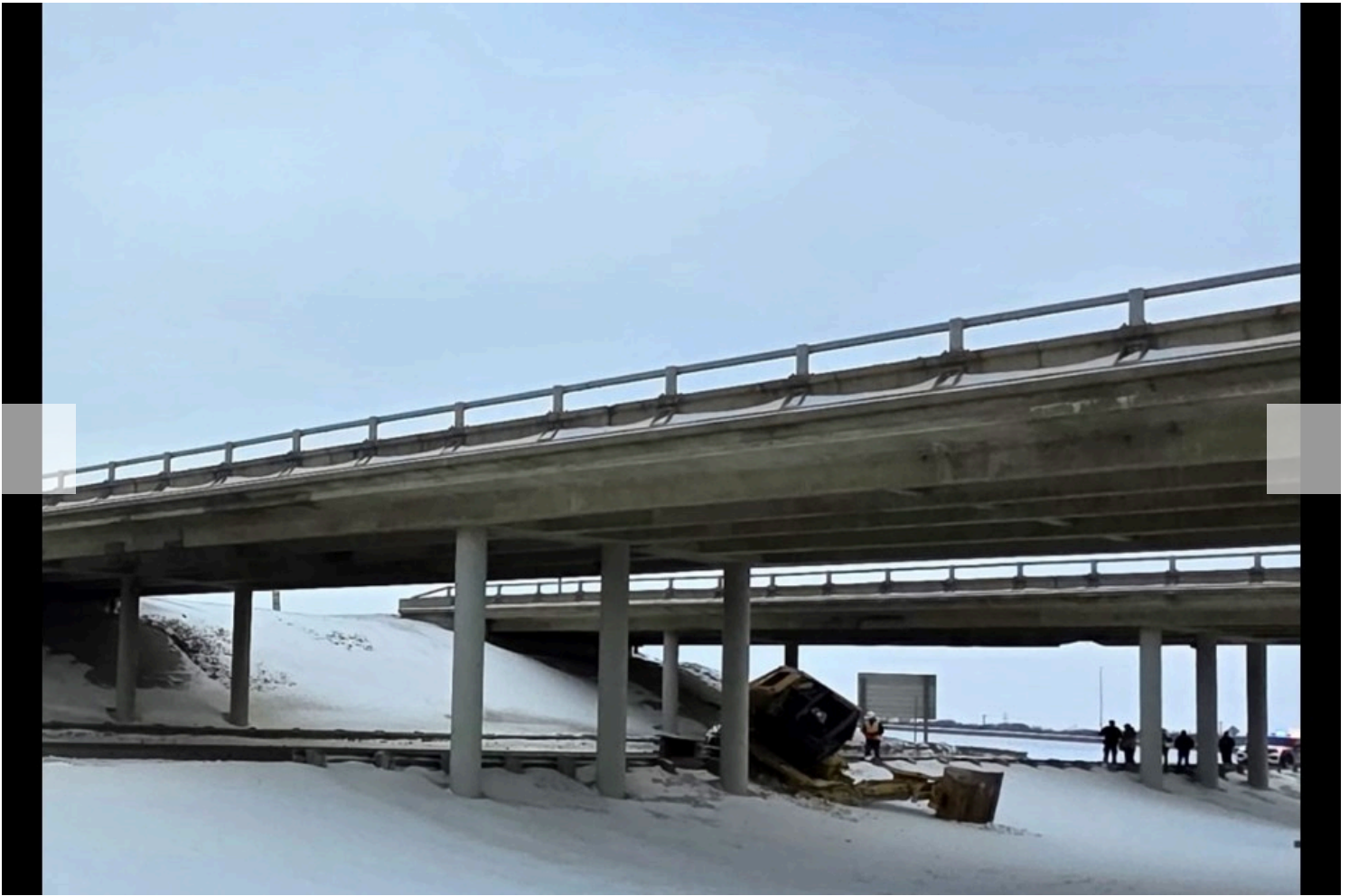
1 / 3 The half portion of the excavator under the overpass. | Jon Perez
