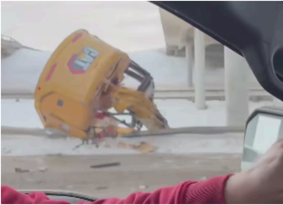
City staff don't yet have a timeline for repairs on the Circle Drive overpass. (Jacob Harmon/Facebook)
